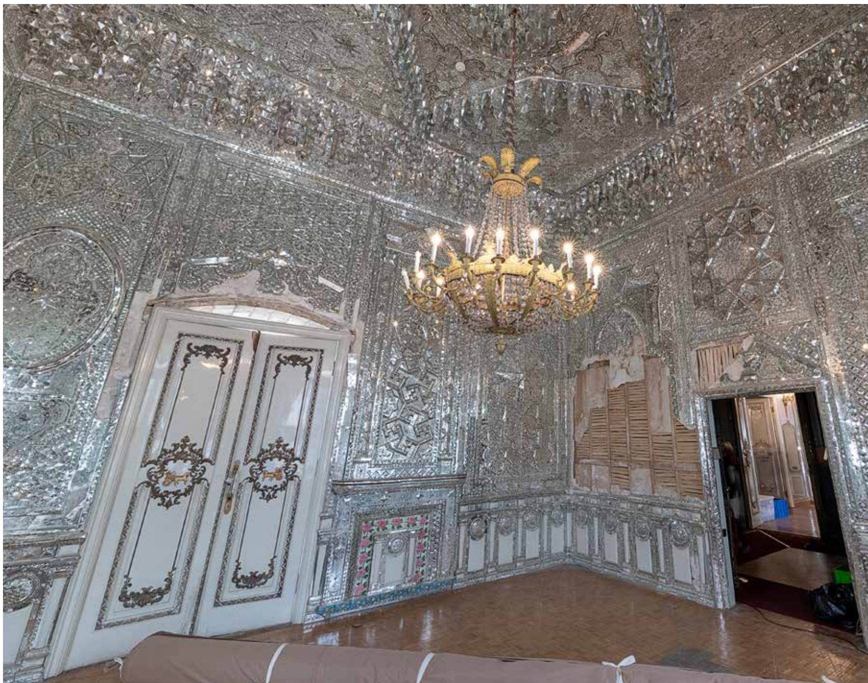
After | The Mirror Hall (Reception Hall) in the Green Palace
