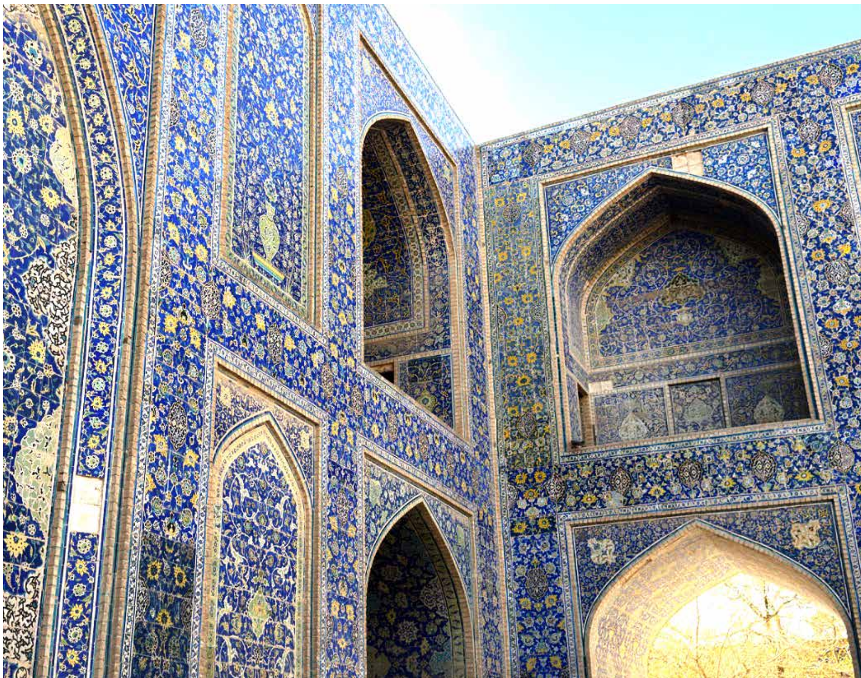
Fallen Tiles of the Imam Mosque of Isfahan
